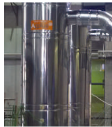
Ensayo vertical Vertical test Essai vertical
